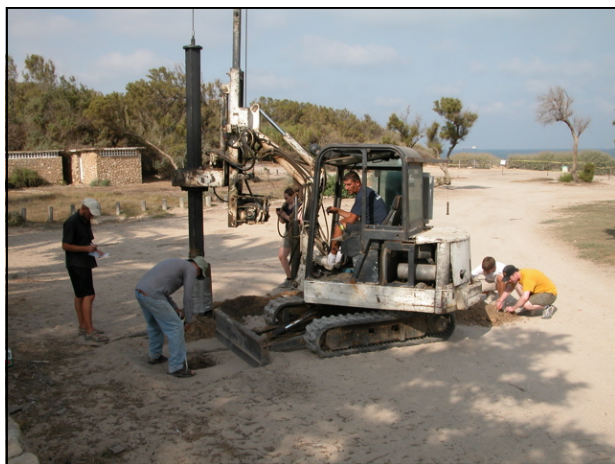
Bucket-auger drill rig at Ashkelon along the Israel-Mediterranean coast, July 2008
